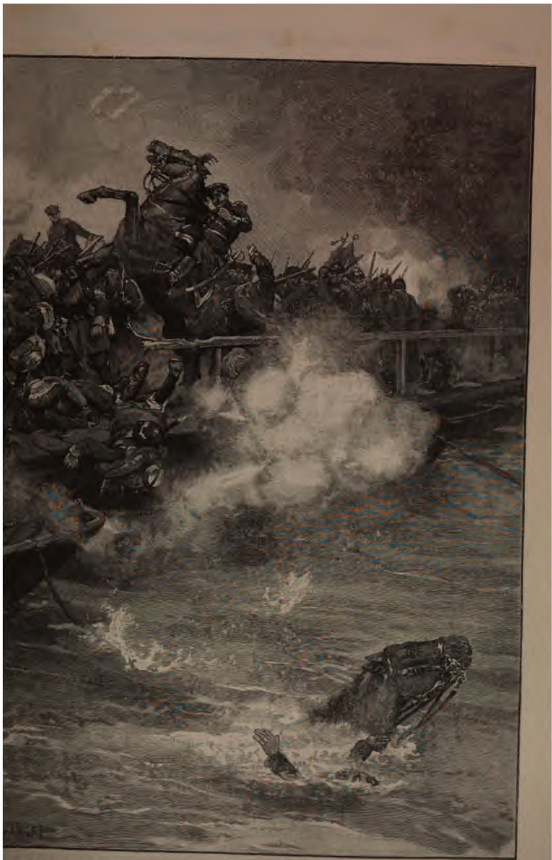
"A TERRIBLE CARNAGE ENSUED UPON THE OVERCROWDED BRIDGE" (A. 464).
